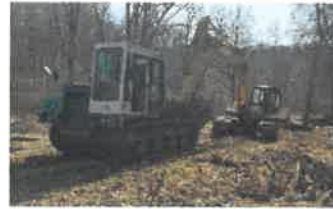
County crews: Cleaning a channel on Bramble Rd., C.R. 37 in Perry Township (left); Excavating an embankment to improve sight distance on Aurora Rd., C.R. 18 in East Township (right)
