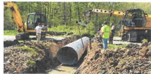
County crews replacing a culvert on Autumn Rd., C.R. 19 near Algonquin Mill in Union Township (above) providing assistance to the County Fair Board during construction of the new show arena (below).
