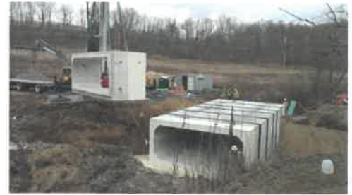
Box culvert installation on Picador Rd., TR 364.
