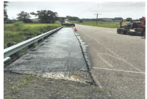
Bridge deck waterproofing Andora Rd., CR 10
